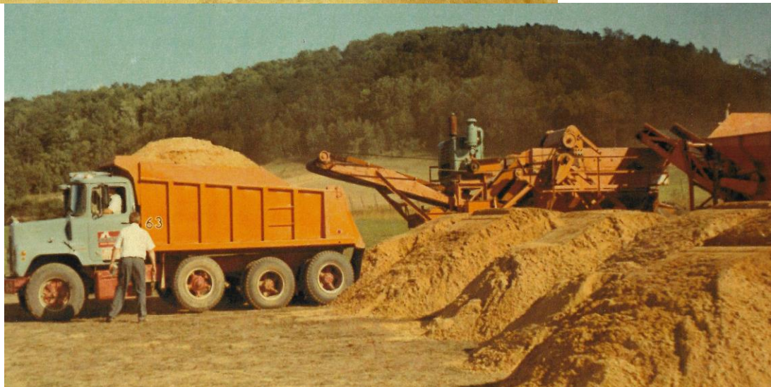
Ralph Soeldner spotting trucks with screening plant in background.
