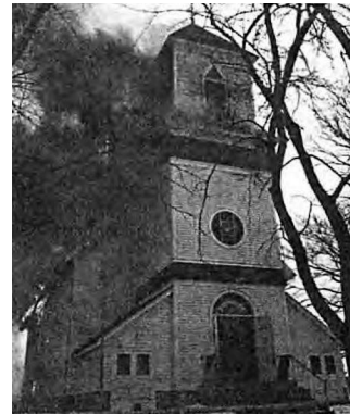
St. Patrick's church fire, Feb. 15, 1962, believed to have started by faulty wiring.
